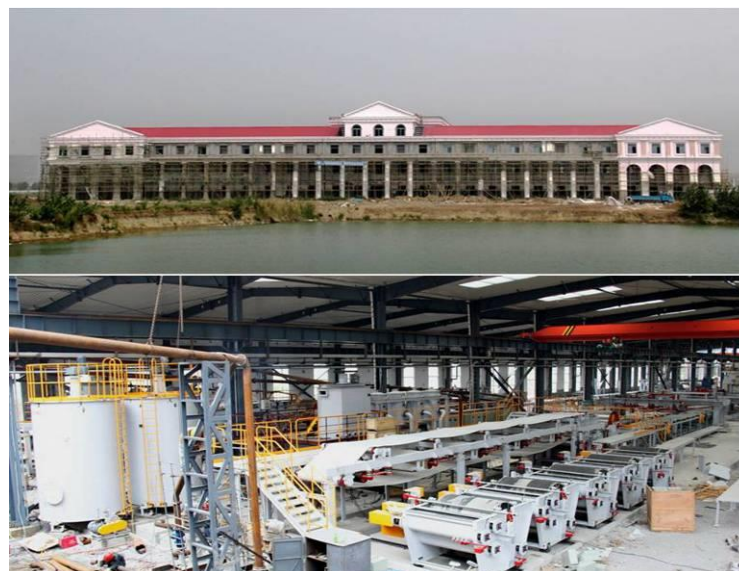
Full view of the engineering construction of Bozhou Conch Venture New Building Materials Company
