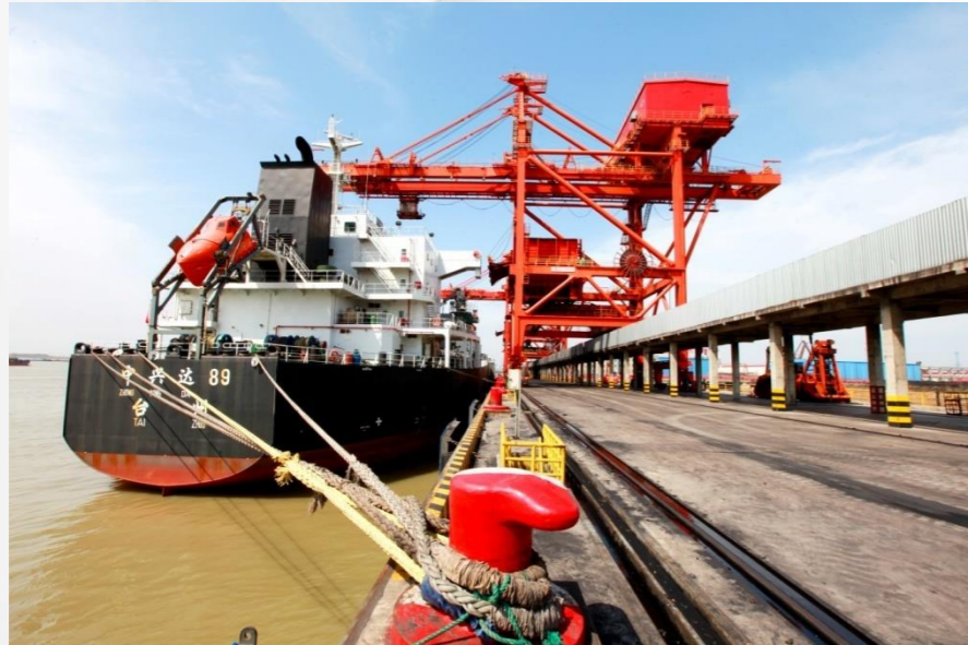
Yangzhou Haichang Port Terminal
