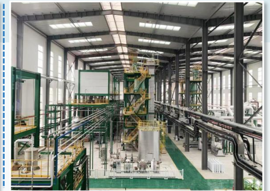
The real scene of the factory building
